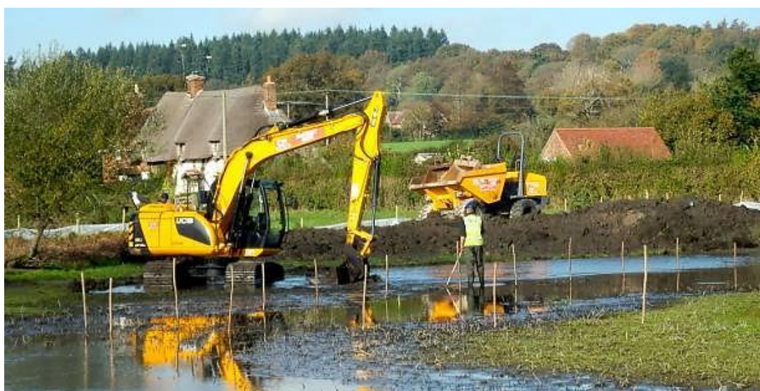
Figure 99: Excavation of Round Pond during 2014 (Photograph: Jo Gore)
