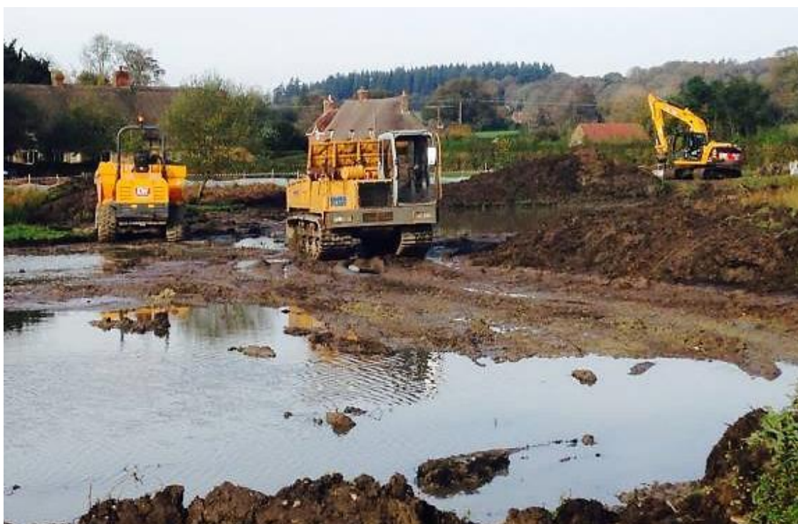
Figure 100: Excavation of Round Pond during 2014 (Photograph: Jo Gore)
