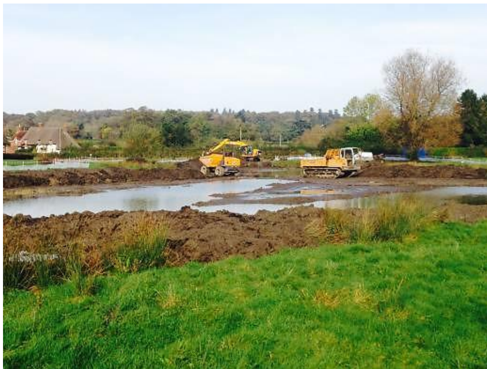
Figure 101: Excavation of Round Pond during 2014 (Photograph: Jo Gore)
