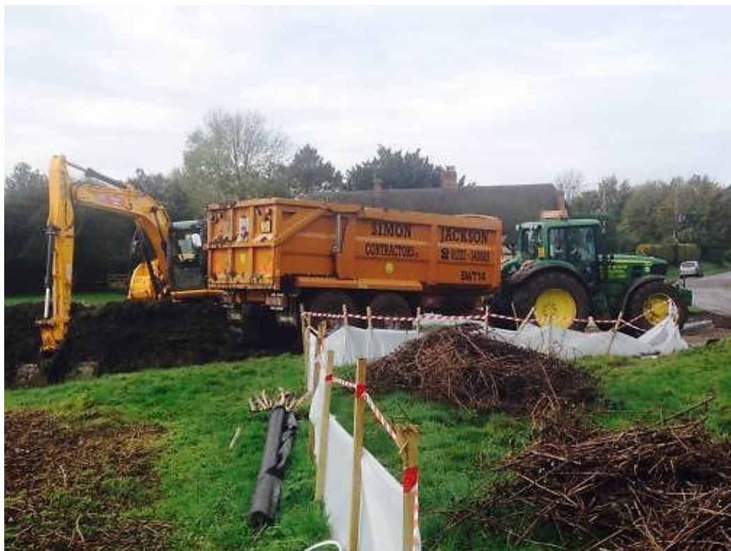
Figure 36: Excavation of Round Pond during Autumn 2014 (Photograph: Joanne Gore)
