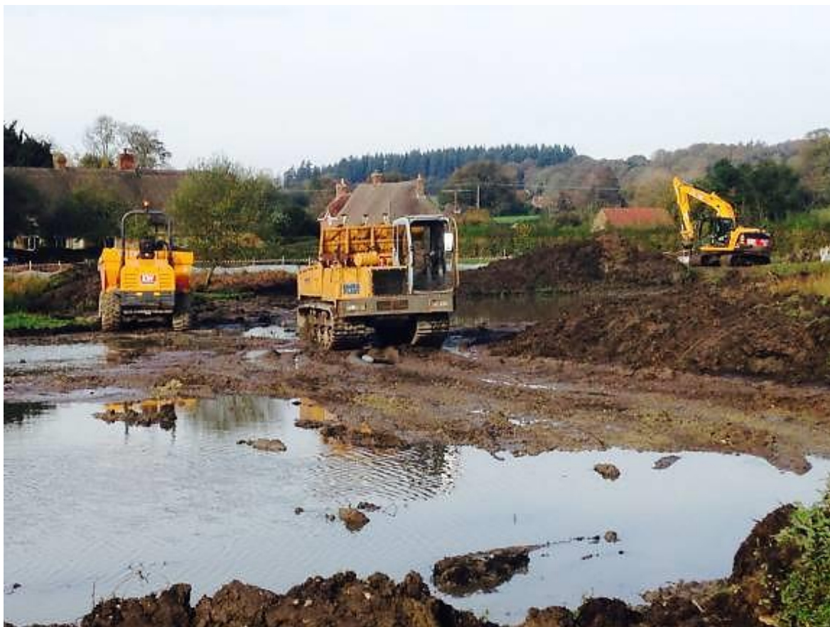
Figure 34: Excavation of Round Pond during Autumn 2014 (Photograph: Joanne Gore)
