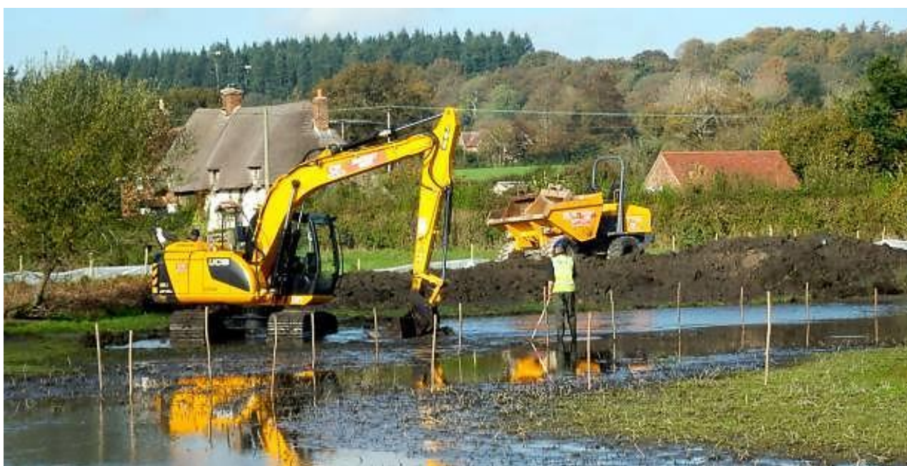
Figure 33: Excavation of Round Pond during Autumn 2014 (Photograph: Joanne Gore)
