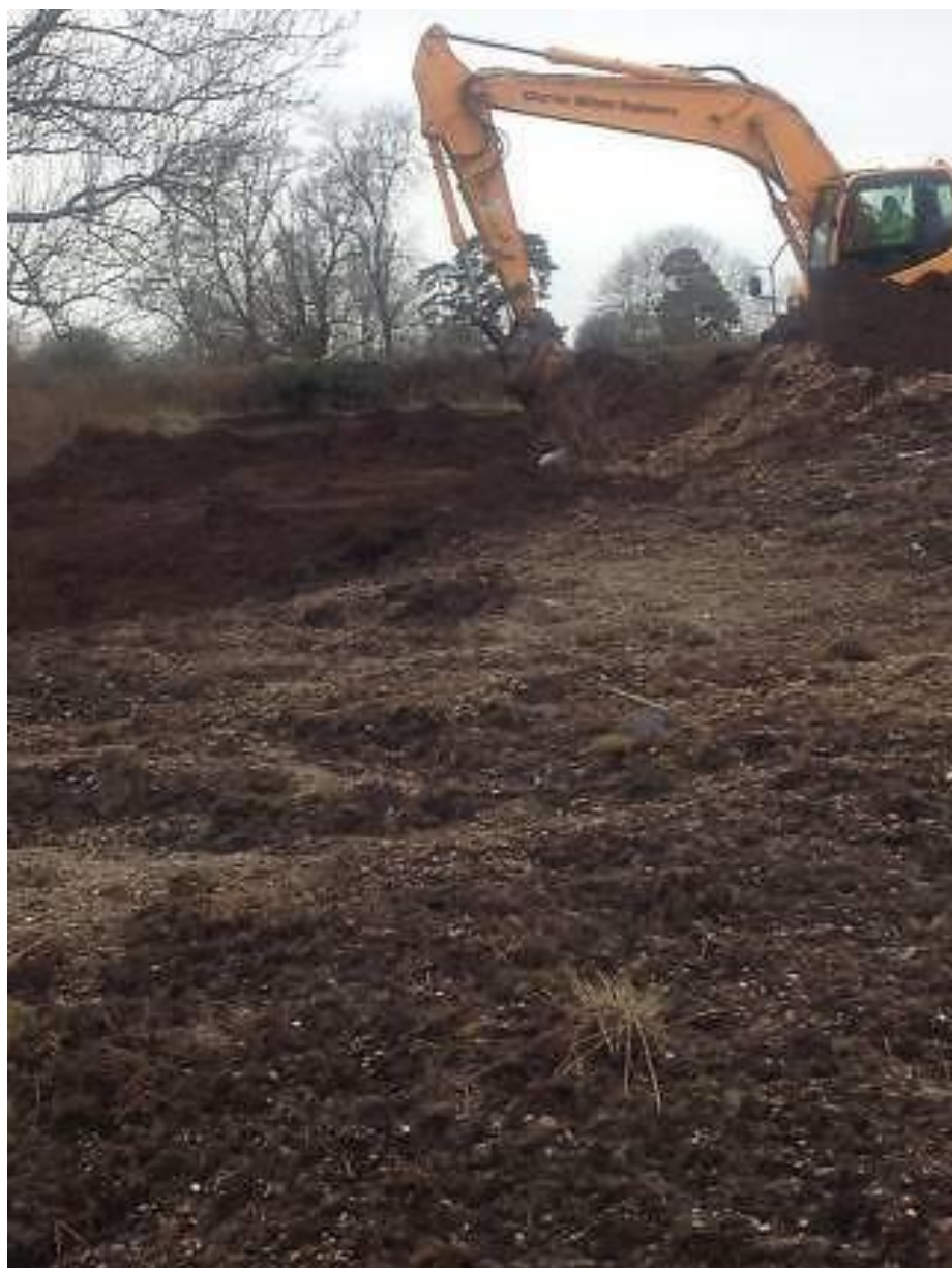
Figure 38: Capping the disposal site during February 2015 (Photograph: Joanne Gore)
