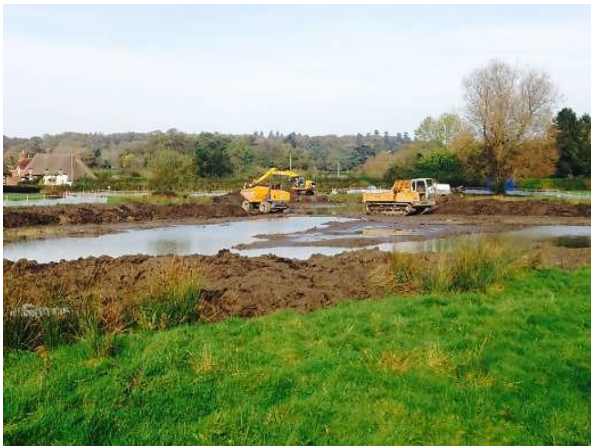
Figure 35: Excavation of Round Pond during Autumn 2014 (Photograph: Joanne Gore)
